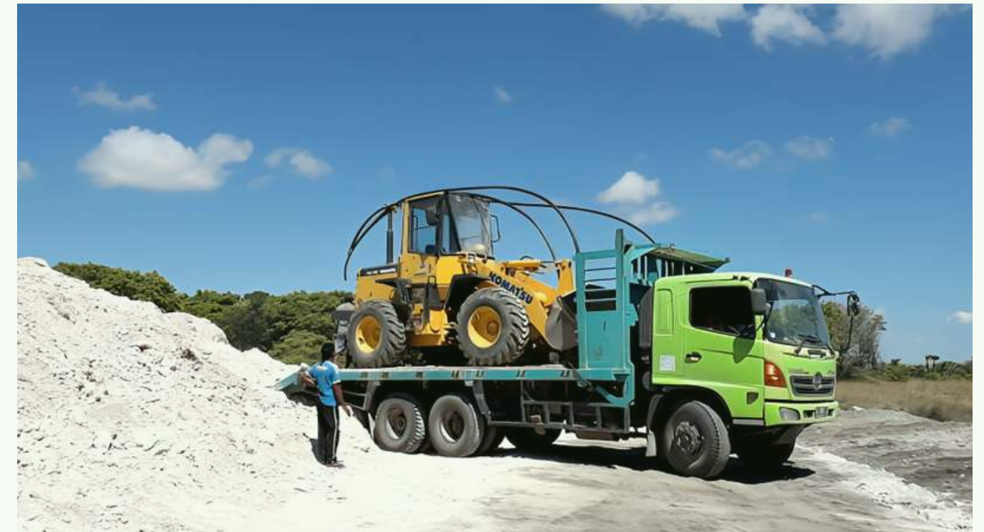
Works for opening the road to Kandora
